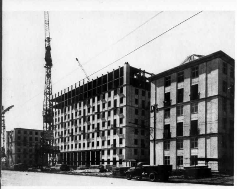
BUILDING SITES ARE BECOMING ASSEMBLY LINES. WHOLE WALLS ARE CONSTRUCTED INDUSTRIALLY AND ONLY NEED ON-THE-SPOT FINISHING. FRAMES, DOORS AND SASHES ARE DELIVERED ALREADY PAINTED AND WITH GLASS IN PLACE. OTHER SECTIONS HAVE A FINISHED CEILING FOR ONE STORY AND A FLOOR FOR THE ONE ABOVE.
