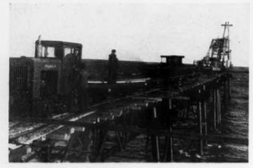
The need for oil keeps bringing new rigs into the system, and this results in extension of the railway trestles further and further into the Caspian Sea.
