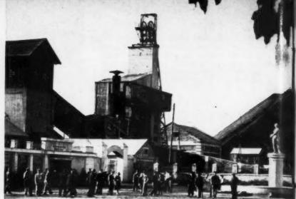
A restored mine in the Donbas. Postwar reconstruction program was not limited to restoration of the wrecked coal industry, a task of tremendous proportions, but dozens of new mines were opened on formerly occupied territory and in other areas. The program also included introduction of many new types of equipment. Today, the nation's coal production is 2.6 times the 1940 level.
