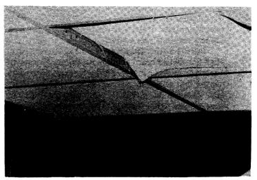
A typical ceiling with loose panels in Newton North High School. Broken panels like this one contributed to the release of asbestos fibers.
