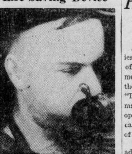
This picture was taken inside the submarine S-4, which was submerged to make deep-sea life-saving tests for the rescue of the crews of wrecked submarines. One of the seamen is shown adjusting a mechanical lung. The invention is only about a year too late, 40 seamen having been killed when trapped in the same S-4 now used in these safety tests.
