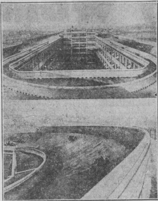
A unique feature of the Fiat automobile plant in Italy is the roof race course on which both racing and stock cars made within the structure are tested. The track is of concrete, with high banked turns, as can be seen from these photos.
