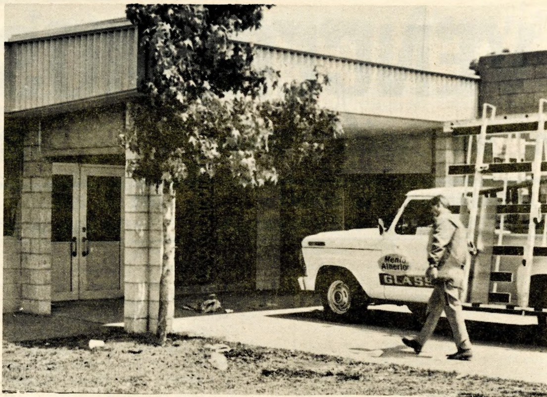
Windows being replaced after the rebellion.
